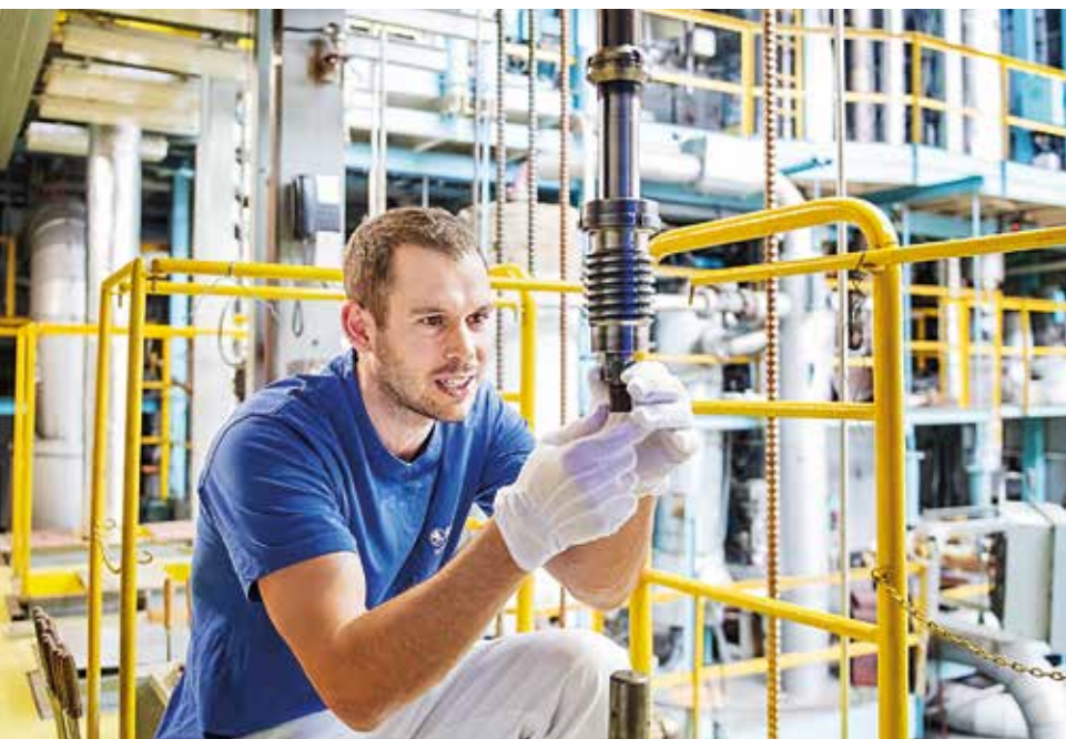
Handover tests of new PRO-M drives
